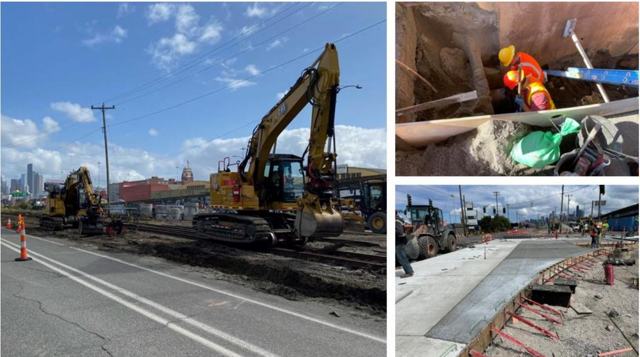
*Clockwise from left: Railroad tracks being removed where the new 2-way protected bike lane will eventually be located; earthquake-resistant watermain pipe installation; new northbound roadway panels on East Marginal Way.*
